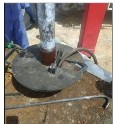
ESP/tubing/cable installation
