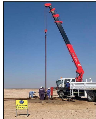
ESP with riser P. pullout
