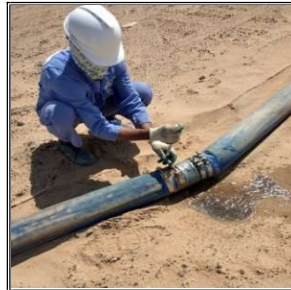
Leak fixing
